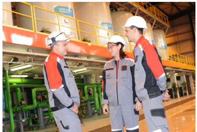
Personal service rooms of the mill have an innovative zoning system arranged
