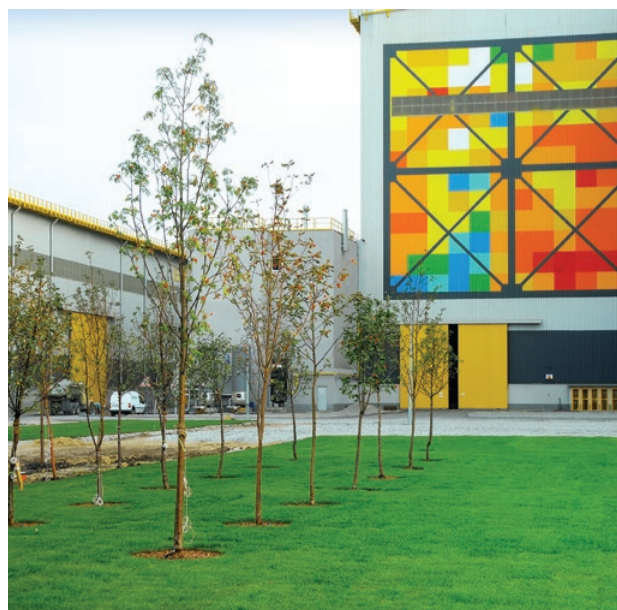
Interpipe Steel – one of the most advanced electric steel-making plants in Europe launched in 2012
